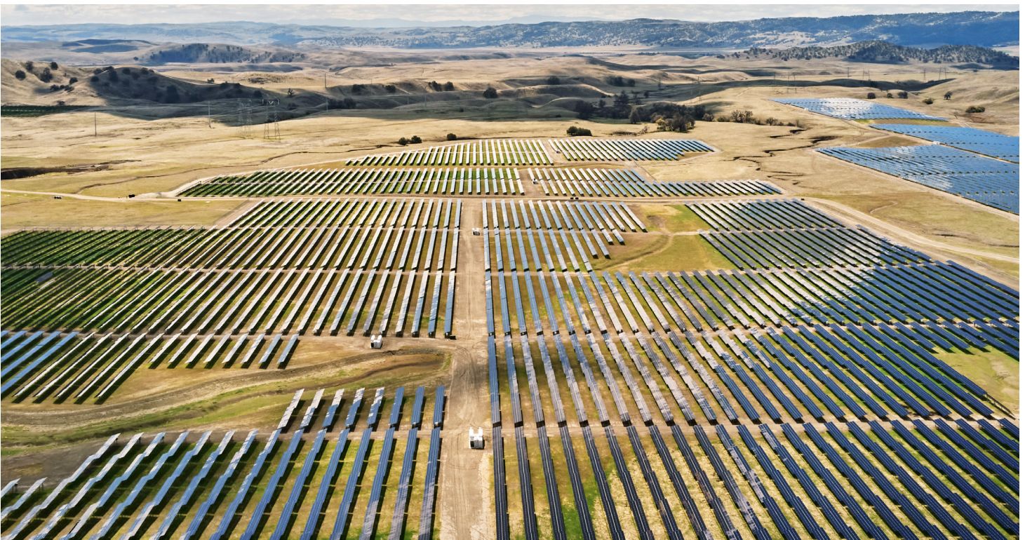
Apple helped create a new utility-scale battery storage project that supports the 130-megawatt California Flats solar farm, which provides renewable energy for our California facilities.
