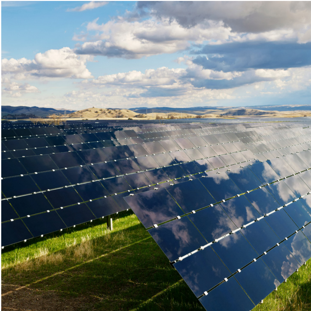
Apple has invested in the California Flats energy storage project, which retains generated clean energy from intermittent renewable sources, including the adjacent 130-megawatt California Flats Solar Project (pictured).
